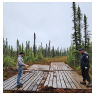
Swamp mats laid to preserve the integrity of the soft soil in areas of high moisture.
